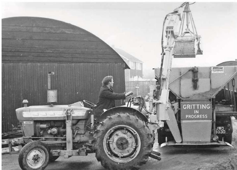
**Left: Turner Engineering modified the hydraulic flail arm from its Hydramower so it could be used for handling bulk materials. Here we see it loading road salt into a gritting lorry using a clam-shell bucket.**
